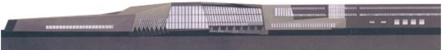
Facing north / Fasade mot nord.
