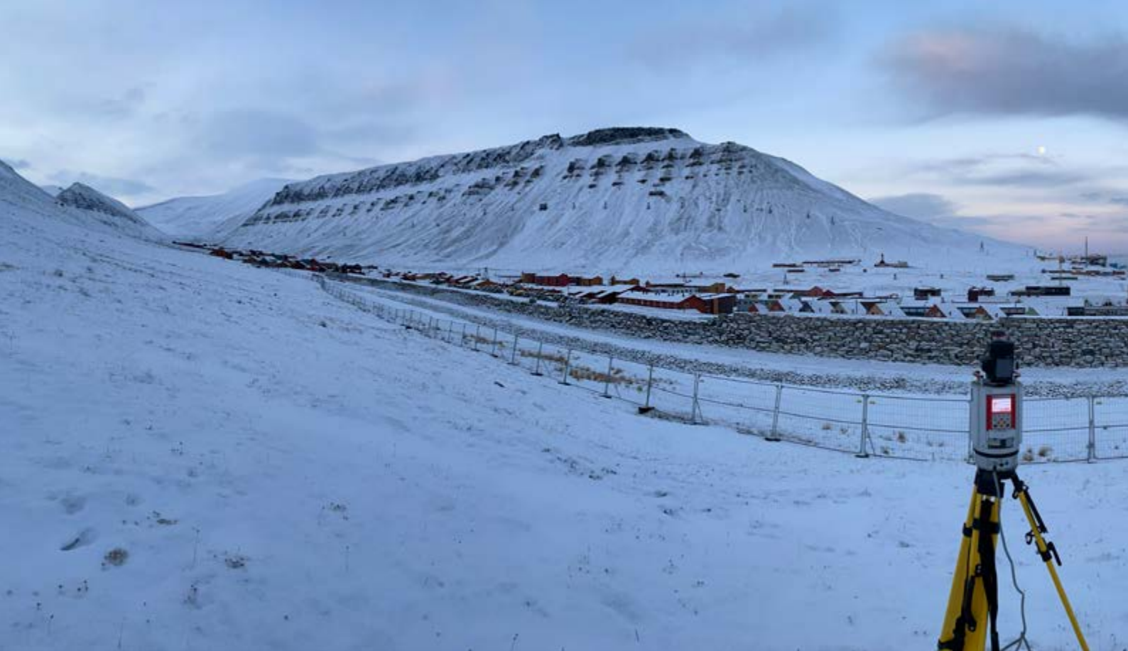
October 2021: Laser scanning is being used to monitor the newly built avalanche protective wall in Longyearbyen. Photo: Nataly Marchenko/UNIS.
