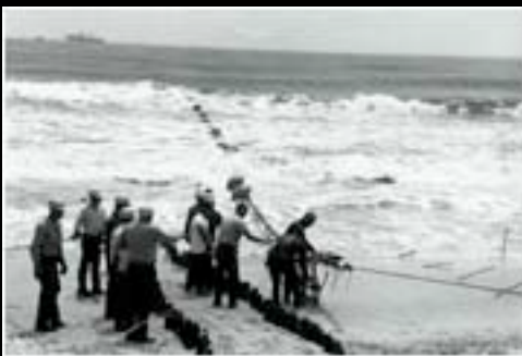
Image about the installation of a sea cable. Figure credit: AT&T.
