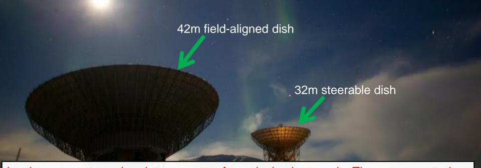
Incoherent scatter radar: detects scatter from single electrons by Thompson scattering
